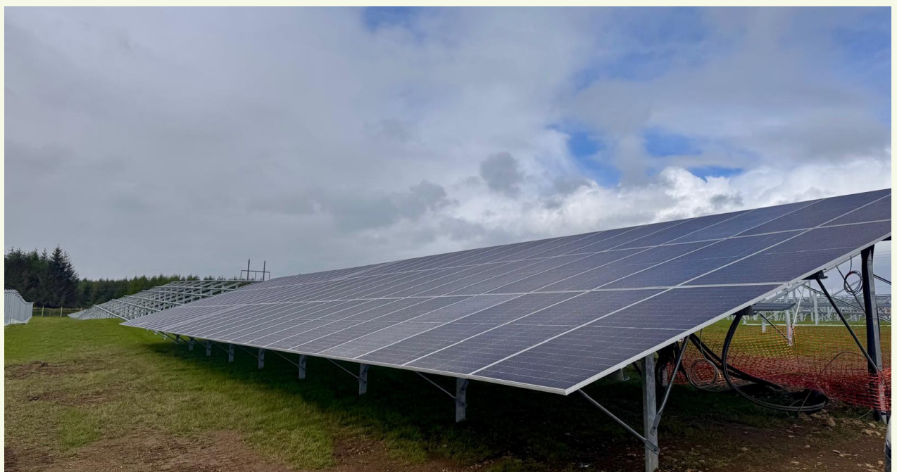
Figure 56: First PV panels installed at Monvallet Solar Farm, Ireland
