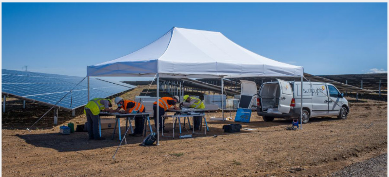
Figure 47: Solar panel inspection and replacement work following drone-based thermography at Poblete Solar Farm, Spain
