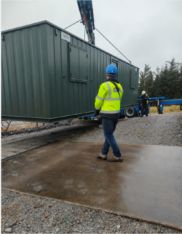
Figure 6: Installation of a new Welfare Unit at Coollegrean Wind Farm, Ireland.
