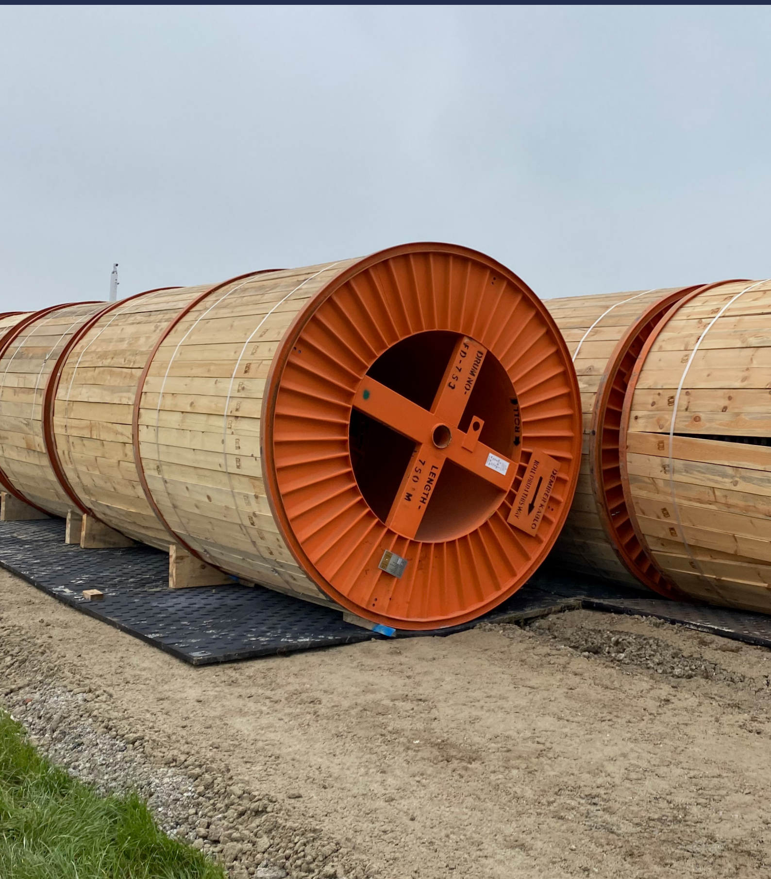
Cables used in the construction of Ockendon 132kV substation/grid connection, England
