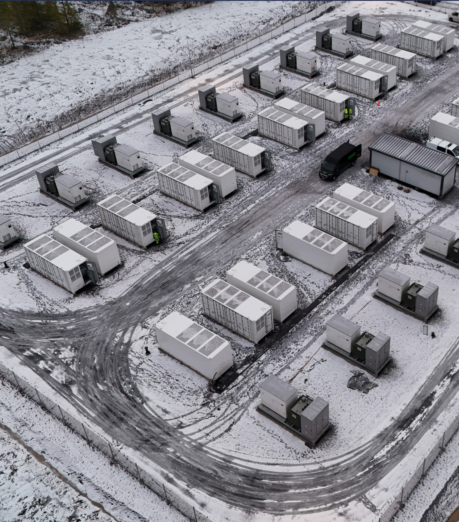
Uusnivala, Finland: 55 MW/110 MWh grid-forming BESS, designed for operation at -40^{\circ}\text{C}
