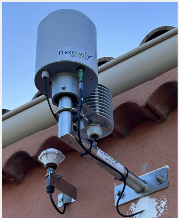
Figure 28: Fleximaus bat protection equipment installed at Provencialis Wind Farm
