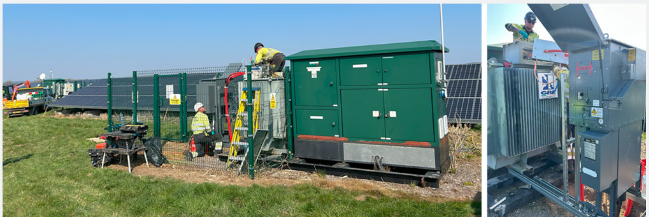
Figure 10: HV improvement works at Brookbarn Apollo Solar site, including the installation of an additional 11kv Circuit Breaker between the site’s two transformer stations
