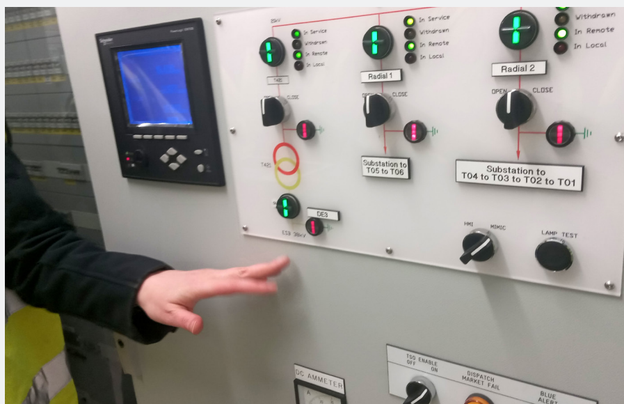
Figure 89: Wind Turbine Switchgear Control Panel
