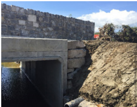
Photo of replaced Drumoscline Bridge, Co. Cavan Ireland
