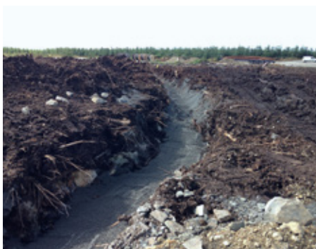
A Trench dug on the Airies site
