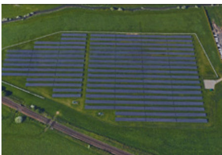
Brook Barn Solar farm
