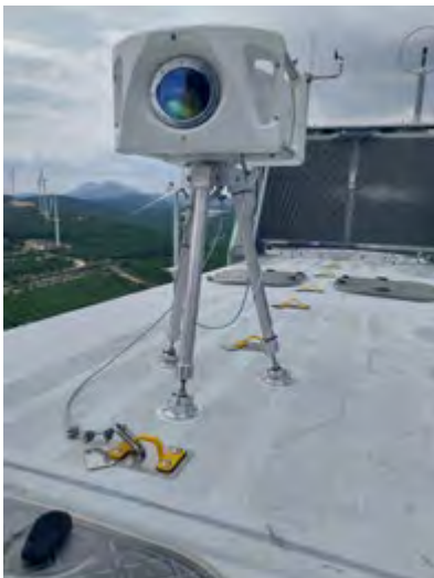
Figure 7: Horizontal LiDAR mounted on turbine nacelle in Provencialis, France
