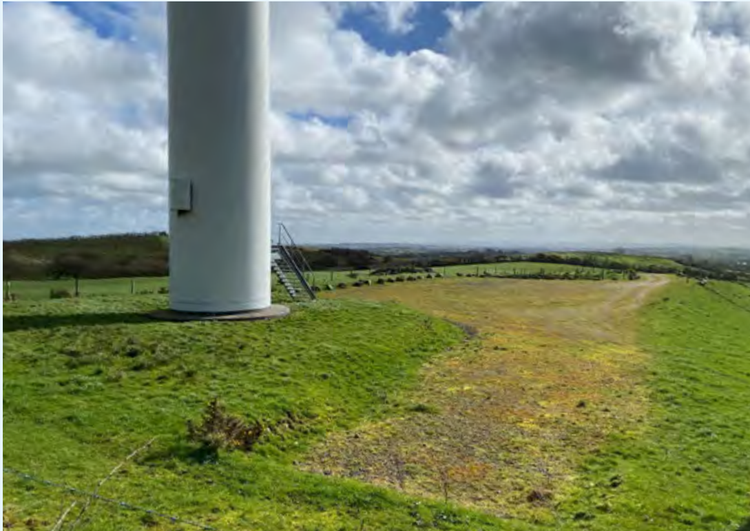
Figure 4: Hardstand rewilding progress on Teevurcher windfarm, Ireland
